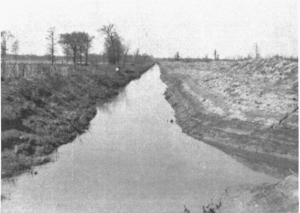
Deep open ditches, or canals, like this one, are used for carrying away large amounts of water in draining extensive areas of swamp land.
