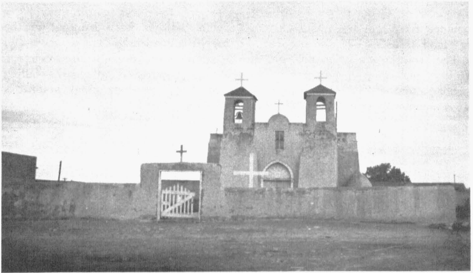
This church, constructed of dried mud blocks and mud plaster, (known as adobe) was built by the early Spanish settlers in the dry climate of New Mexico over 175 years ago. In Missouri the rains would have melted it down within a year or two.
