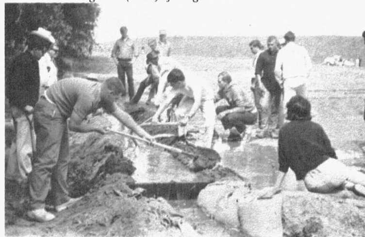
▼ Patching buns (dikes) of irrigation ditch.
