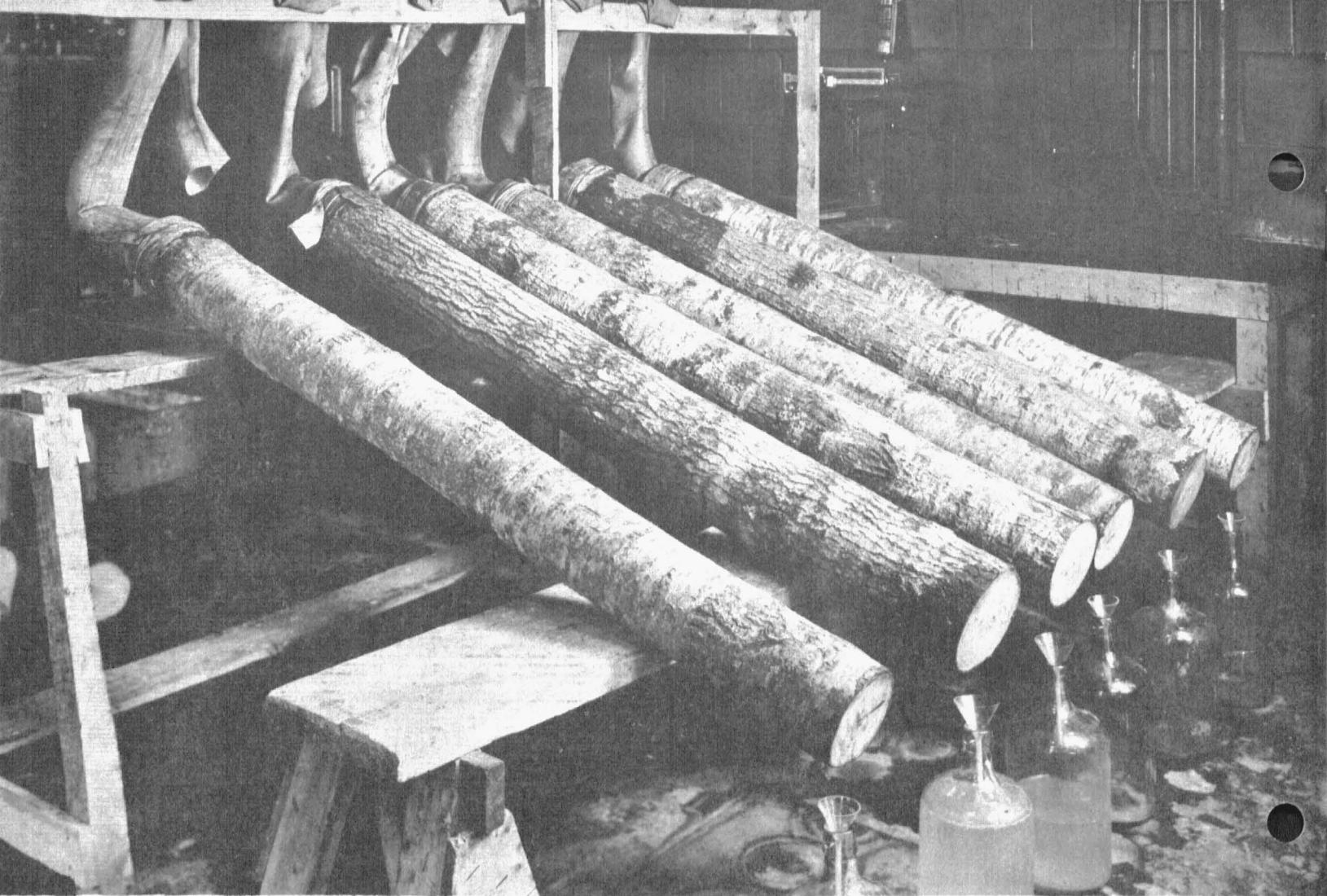
Fig.2. Treating posts with zinc chloride by the tire tube method. (Photo by U. S. Forest Service.)
