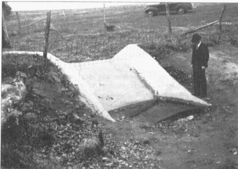
Fig. 10.—This Missouri dam carries water from approximately 30 acres of terraced land. The water comes to it through a broad constructed grassed outlet 34 feet wide along the field boundary to the left. Notice the water standing in the stilling basin below. The velocity check which is here submerged has prevented the discharge flow from scouring out the channel of the main drain below.
