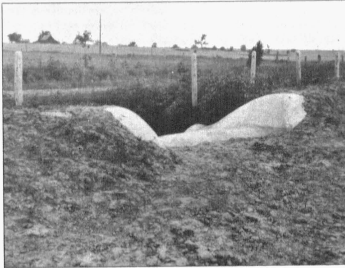
A Missouri soil saving dam in place, with wings covered by the backfill and earth puddled-in to the approximate level of the notch.
