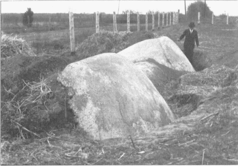
Fig. 6.—The upstream side of a dam in Boone County with the structure completed except for the earth backfill. Notice the low portion in the center known as the "notch", which will carry the water over the structure. The wings are to be covered with earth and a small terrace like dyke is to be placed along the fence to divert water through the notch.
