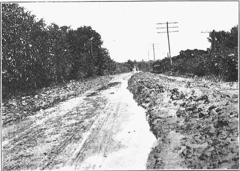
Fig. 3. Opened with Road Scraper
