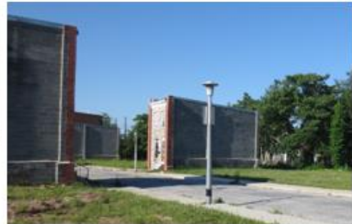
Figure 7. “Missing tooth” vacant lots (dark gray) with an example of two – three missing rowhomes in Carrolton Ridge (top) and extensive missing tooth vacant lots surrounding one remaining rowhome in South Clifton Park neighborhood (bottom).
