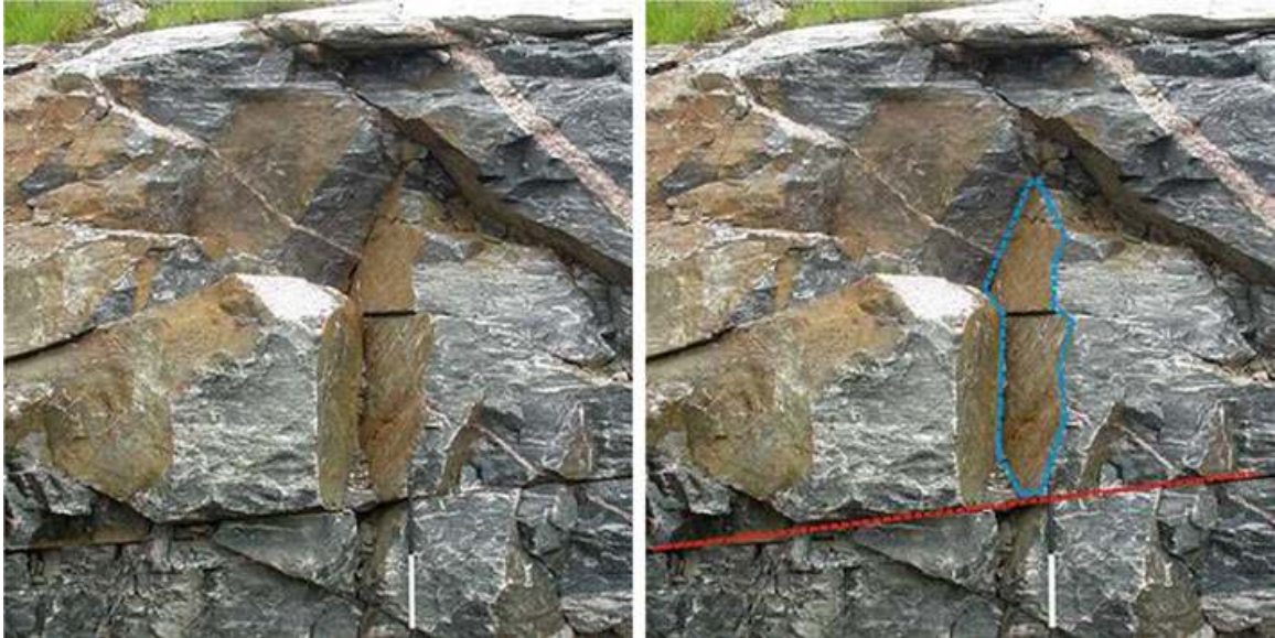
Figure 7.8: Rock cut containing both fracture traces (red line) and facets (cyan polygon) [13].
