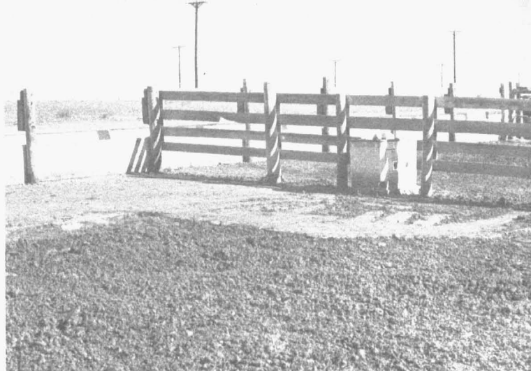
Automatic waterers were placed on the center line of each lot and concrete paving was extended around them.
