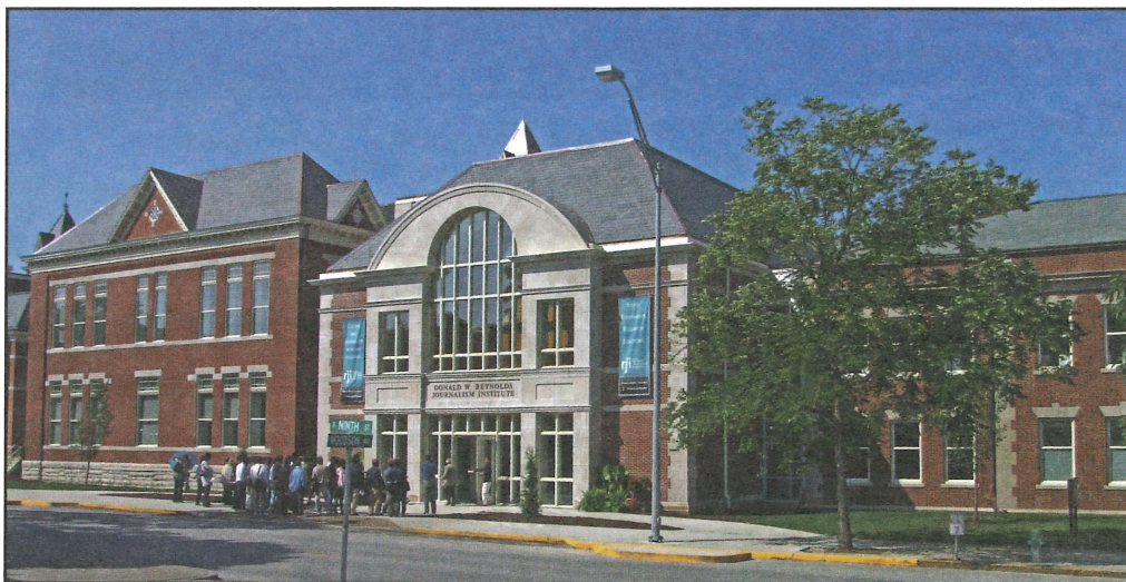
The Donald W. Reynolds Journalism Institute project renovated two historic buildings – the Sociology Building and Walter Williams Hall – and built a connecting addition to house modern media technology.
