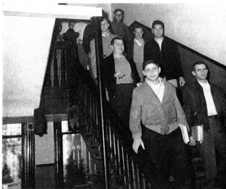
The pipe in center supports a brace for a stairway in the B&PA Building. The heavy student traffic puts a burden on the wooden stairs.
