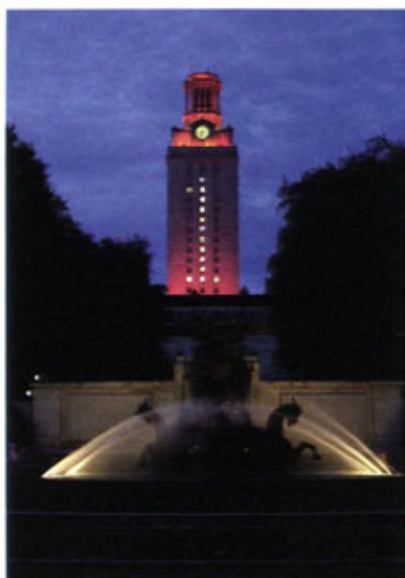
See Austin on a Mizzou football weekend tour as the Tigers play the Longhorns. This tower anchors the University of Texas campus.
