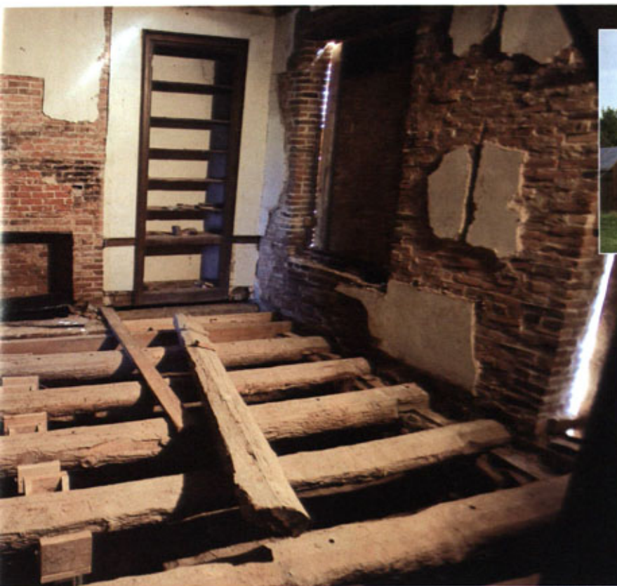
Workers are rehabilitating the circa 1821 Hickman house in New Franklin, Mo., at MU's Horticulture and Agroforestry Research Center. The floor joists are logs leveled at the top.
