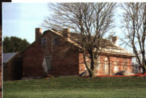
Workers are rehabilitating the circa 1821 Hickman house in New Franklin, Mo., at MU's Horticulture and Agroforestry Research Center. The floor joists are logs leveled at the top.
