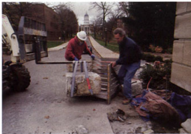
John Kruger, left, of Mid-Continental Restoration Co. of Ft. Scott, Kan., and Ed Drane, contract manager for MU Planning and Design and Construction, slide a wooden pallet under the suspended cornerstone. It was removed from the gate and will be relocated in Jesse Hall.
