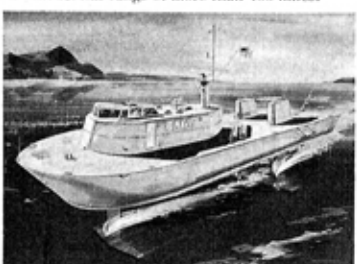
Drawing of 115-foot hydrofoil craft Boeing is building for U.S. Navy. Riding out of water, craft will "fly" at speeds up to 45 knots on underwater wings.
