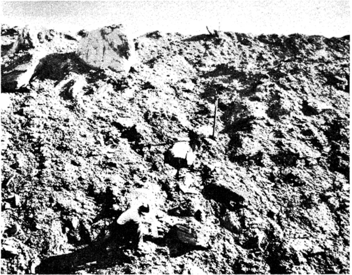
Figure 4.—Eighteen-month-old bank, Crawford County, Kansas, created by electric shovel mining the Weir, No. 6, coal. The surface is composed of 17 per cent soil-sized particles, 2 mm. or less in diameter; 39 per cent larger particles, 2 mm. to 2 inches in size, and 44 per cent, 2 inches and larger.
