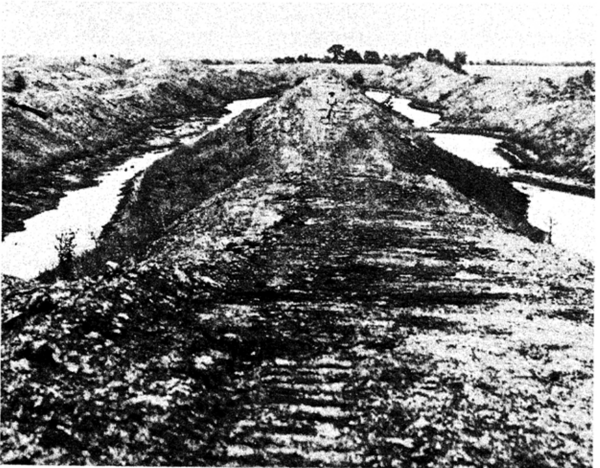
Figure 12.—New pasture project on Mineral, No. 9, coal banks in Cherokee County, Kansas. Access roads have been constructed by striking off the tops of the ridges with a bulldozer. The area will be seeded with lespedeza and sweet clover.
