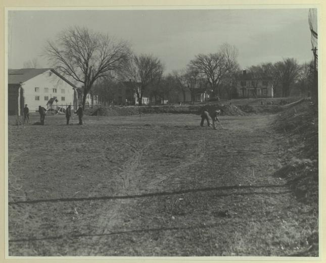
This picture shows workmen preparing to raise this group of tennis courts to a level with those on the extreme right in the picture, which are several feet above these on which work is being conducted. This improvement is going on back of Rothwell Gymnasium.
