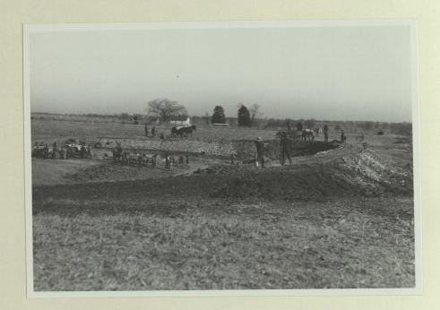
This photograph shows the further renovation of the Dairy Department's pond on the college farm. Those engaged in the project are here shown throwing up dirt for the dam and excavating for the reservoir which will hold the water.
