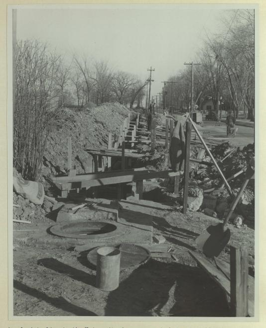
An electric line to the University farm campus is being installed to replace an old line which was unsafe. The picture shows part of the overhead line to the left in the distance. Part of the steam trench, described on the following page, also is shown.
