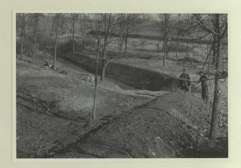
Excess water during rains proved to be a source of much annoyance and some damage to soil by erosion, but this will be ended by a pond now being constructed on Turner Station farm. This project will eliminate costly loss of soil by erosion and the needless appearance of small clefts in the soil following a heavy rain. The photograph shows part of the work being done by C.W.A. men.
