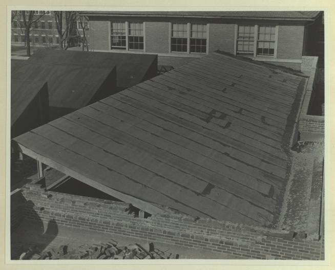
A roof has been placed on the heat treating laboratory and storage room of the Mechanical Engineering shops. This photograph shows the completed job, the earlier stages of which were shown in another photograph. This improvement is part of reconstruction of engineering shops. This renovation will allow the shops to be moved into the building next to the Engineering Building, and is part of the plan to unify activities of the College of Engineering.
