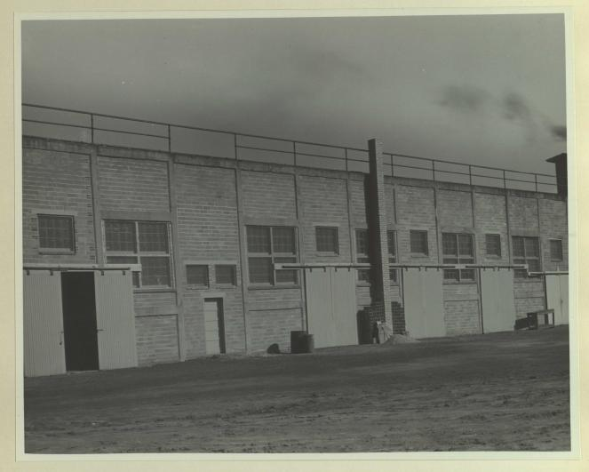
A fire hazard was removed and storerooms for equipment of the field artillery greatly improved when space under the bleachers at Rollins Field was reconstructed and decayed wooded members replaced by brick and concrete.
