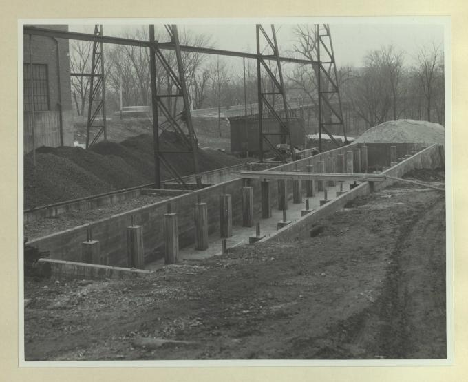
Greater efficiency and less cost is expected of the 600 kw. turbine generator to be served by the cooling tower being added as improvement to the University power plant. The picture shows the basin and foundation for the cypress superstructure which will rise above the basin. The tower will cool the circulating water from the condenser of the 600 kw. unit. Water will spray through the nozzles at the top of the tower, releasing the heat absorbed in condensing the exhaust steam from the turbine.
