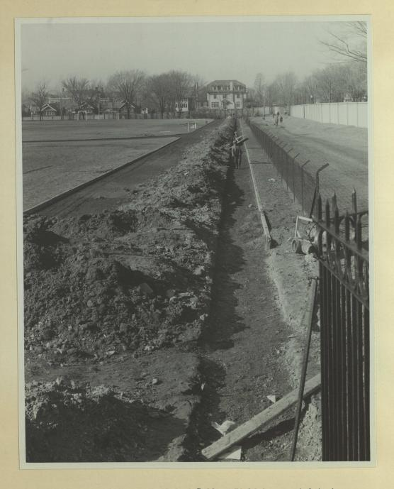
A drainage system being installed at Rollins Field is expected to improve greatly the condition of the cinder track. Heretofore the track frequently was flooded with water every time it rained, leaving it soft and in a poor condition. Often it was out of shape for important track and field contests. The new tile drain will relieve this condition.
