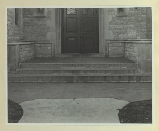
A solid foundation was placed underneath the northwest porch of Waters Auditorium, and the outside balustrade was reinforced. The structure previously suffered much deterioration from cracking as the stonework settled. Had this not been repaired, the porch would in time have become unsightly as the stone and mortar broke loose from fastenings.
