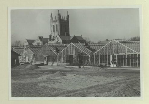
The decay and state of disrepair will disappear from the University greenhouses when improvements now under way are completed. Much of the framework was in a bad state and part of the structures was in danger of damage by wind blowing on weakened members. The work will strengthen the framework and make the buildings more attractive.
