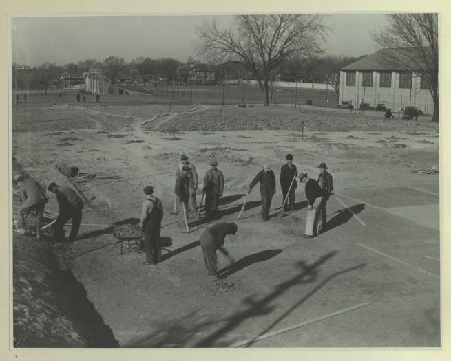
A gang of workmen cut a two-foot grade from the east to insure proper drainage of this set of tennis courts back of Rothwell Gymnasium. This drainage will enable students to play on all of the courts, instead of having to wait unnecessarily long for water to drain from some of them.
