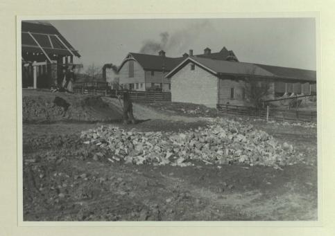
The photograph shows part of the C.W.A. work being conducted on the farm campus. The lot is being graded and a rock foundation laid for an improved road leading to the buildings. Prior to the improvement, the lot was unsightly, uneven and did not have proper drainage. The illustration shows the benefits which will be derived when this project is concluded.
