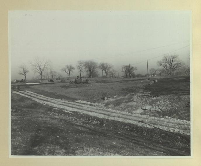
The photograph shows construction work being done on the road leading from the R.O.T.C. stables to Memorial Stadium. This road formerly was uneven, frequently muddy and difficult to traverse much of the time. The improvement connects the south end of the stadium with the main road leading to the spectators' west entrance.
