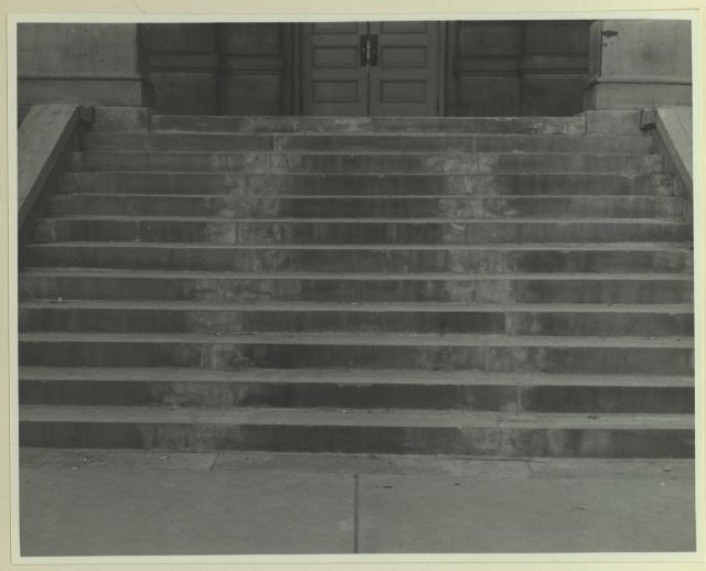
South steps of Jesse Hall were treacherous because of ridges worn on the edges by countless passage of students' feet. This condition was particularly dangerous in wet or freezing
