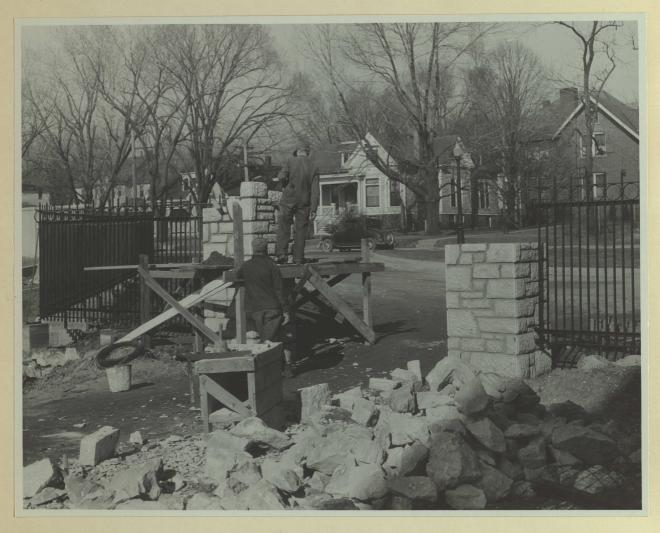
Workmen are shown in the picture constructing a gate to Rollins Athletic Field at the University. The structure will be of stone and will be next to the Field House. This is a greatly needed improvement, for heretofore no provision was made to lock the field except by an antiquated, sagging gate, or by chain or other improvised and unsightly means.
