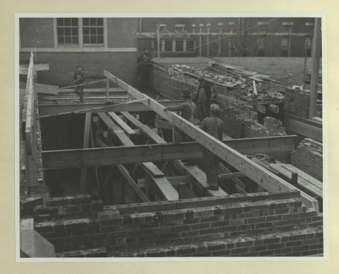
Roofing and Flooring for a formerly open and disused structure will provide the new home for the engineering shops which now will be in the Mechanic Arts Building. This centralizes this work, making it possible for closer supervision in this department. This improvement also will add to the appearance of the Mechanic Arts Building and its appenditures. The picture shows the superstructure with a crew engaged in renovation.
