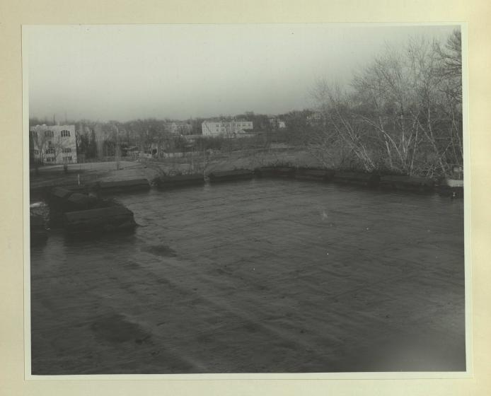
The same situation existed on the cast flat deck of Rothwell Gymnasium as did on the west side, with a constant stream of water leaking through to the floor below every time it rained. The new roof will eliminate this exasperating condition.
