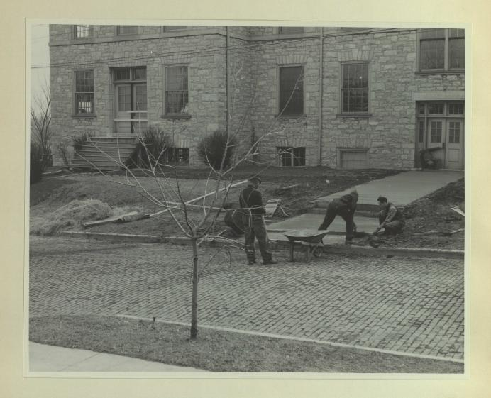
A concrete sidewalk replaces the mudhole which formerly led from the street to the front entrance of the Veterinary Building. The former thoroughfare from Bouchelle to the entrance was both unsightly and a mire which was difficult and uncomfortable to transverse in bad weather. It also was an unsightly and incongrous appendage to what otherwise is an impressive building.
