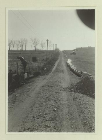
Destruction of the roadway and culvert by flood waters in the Animal Husbandry pastures will be at an end when the drainage tiling alongside the roadway is completed. Heavy collection of water during the rainy spells caused much damage by erosion and washing. Workmen are shown laying the tiling.
