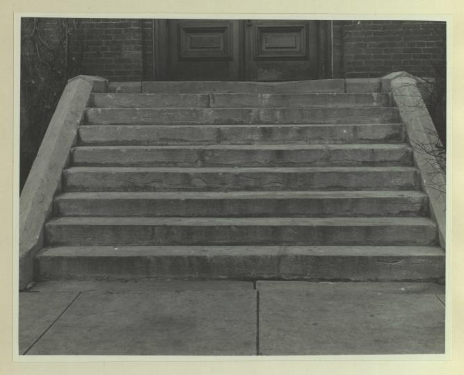
East steps of Switzler Hall were in the same dangerous condition as those at Jesse Hall, but possibly this was more aggravated in the former case. Picture shows creases and cracks on under side of stone steps after they were turned over. These unsightly and rough edges were on top before the surfaces were reversed, and hindered movements up and down the steps.
