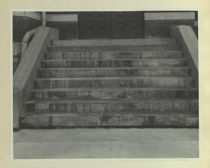
The south entrance to the Old Chemistry Building was a fire hazard because the doors opened inward from the steps. The building had an inadequate landing, making it difficult to change the doors. The structure is old and decidedly not fireproof.
