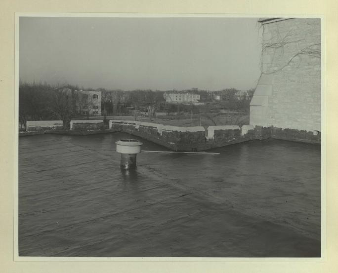
Much annoyance, cost and trouble was eliminated when a new roof was placed on the west flat deck of Rothwell Gymnasium. The old covering leaked and allowed water to drip to the floor below. This work was needed for many years before finally completed.
