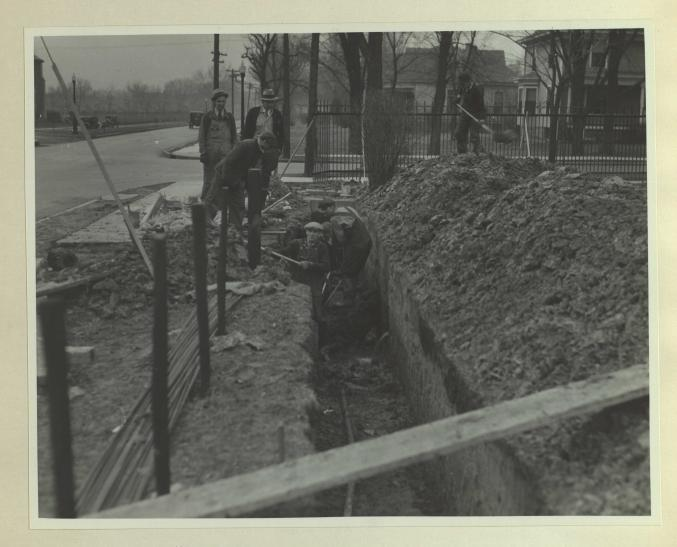
Cost of providing heat to the University farm buildings will greatly decrease and much smoke abatement will be realized as a result of constructing a concrete trench to house steam pipes running from the central heating plant to the farm buildings. When steam pipes are installed, the farm heating plant will be closed. This plant is expensive to operate and is a neighborhood nuisance because of smoke and ashes which come from it. The picture shows workmen constructing the trench.
