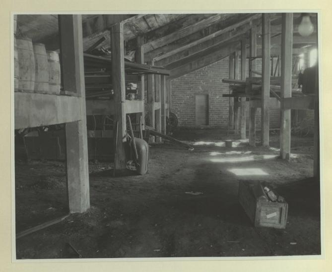
A concrete floor will replace the old soggy and evil-smelling surface of the field artillery storeroom under Rollins Field. The hard-surface floor will enable heavy army equipment to be moved with greater ease than formerly and will help protect it against rust and dirt.
