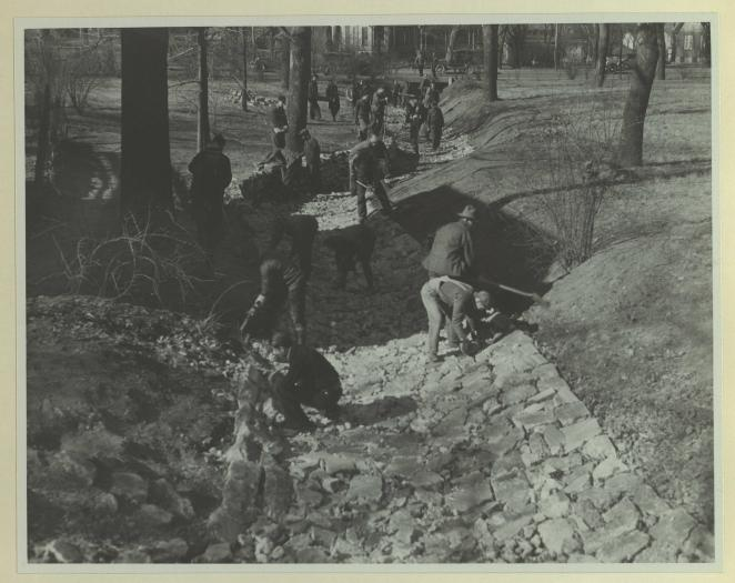
A more attractive and less turbulent stream will flow through the channel on the West Campus during rains, after workmen complete wrapping the bed with broken stone. Formerly, the stream was muddy, dirty and often the seat of insanitary mudholes which remained after surplus water should have flowed away following rains.
