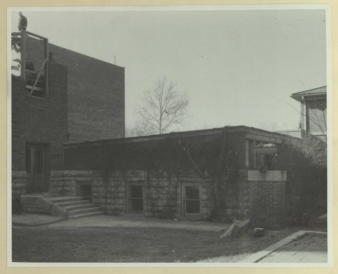
The southwest wing of the Mechanic Arts Building is being reconstructed for the first time since the fire of 1911, which will be a marked step in unifying the engineering department. The northwest wall of the structure is under construction. The larger wall is seen in the background. It will rise about six feet higher before it is completed. The roof is expected to be completed about the middle of February or a little later.
