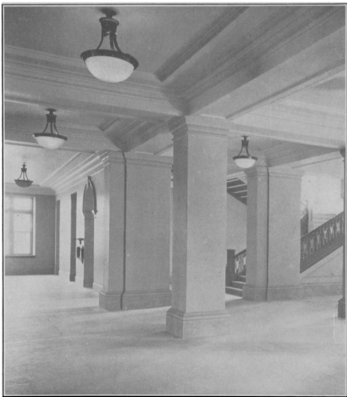
Entrance lobby and east stairway
