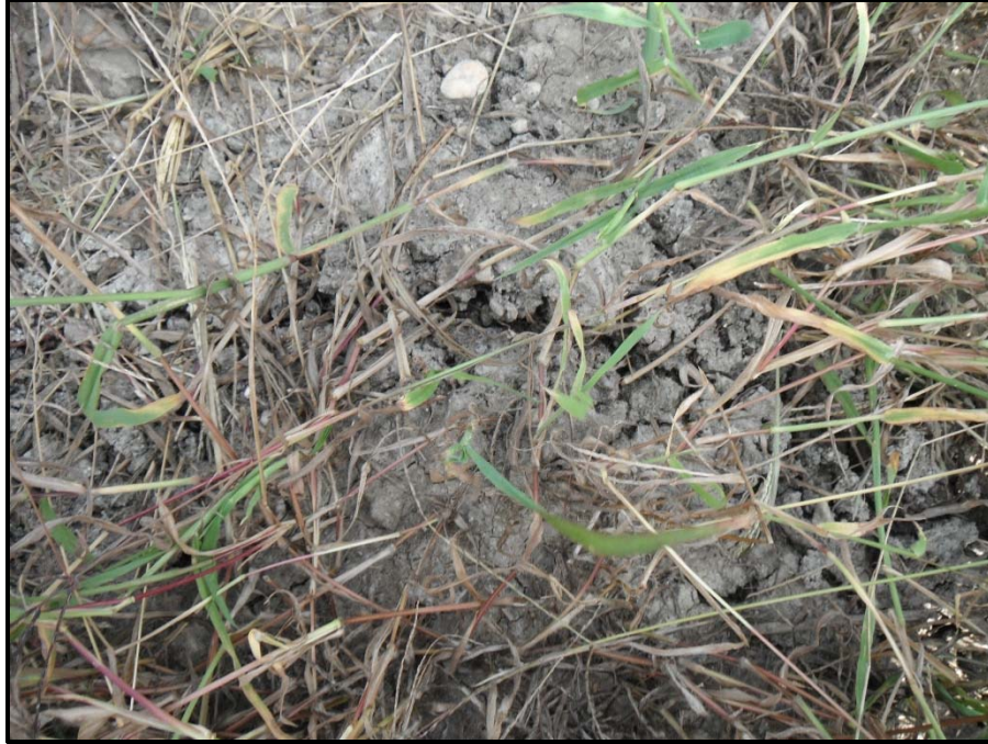
Figure 5.34: Tension Crack near Installed Soil Moisture Sensors at McBaine, MO Field Site
