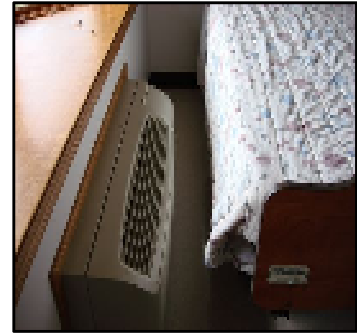
Figure 25. Facility # 1 Temperature Control
