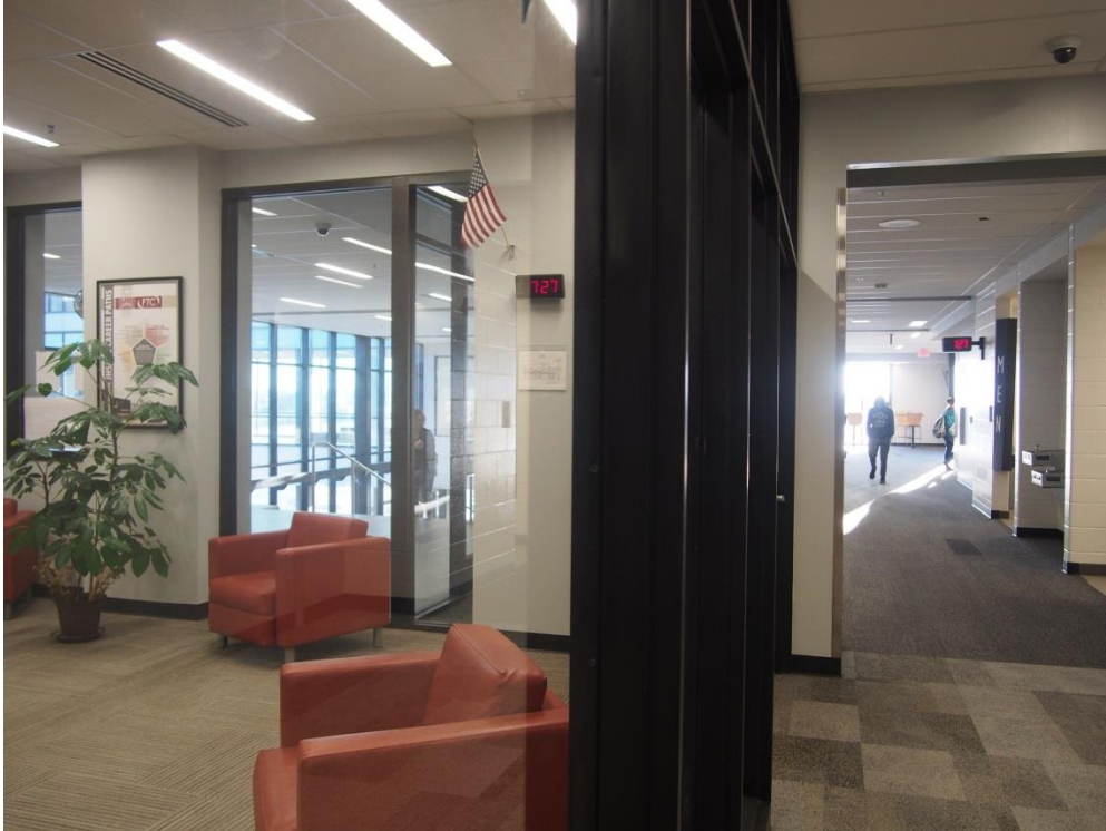
Figure 45. Interior window wall between one assistant principal's office suite and the hallway lobby on the second floor
