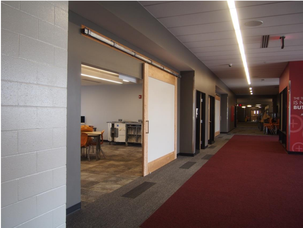
Figure 27. Sliding barn doors between classrooms and hallways
