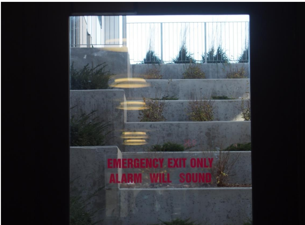
Figure 28. Door to the courtyard
