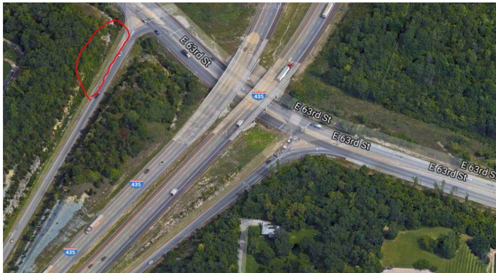
Figure 2.5. 63 rd street section location along the ramp to southbound Interstate 435 (63 rd H) circled with red line. Kansas City, MO.
