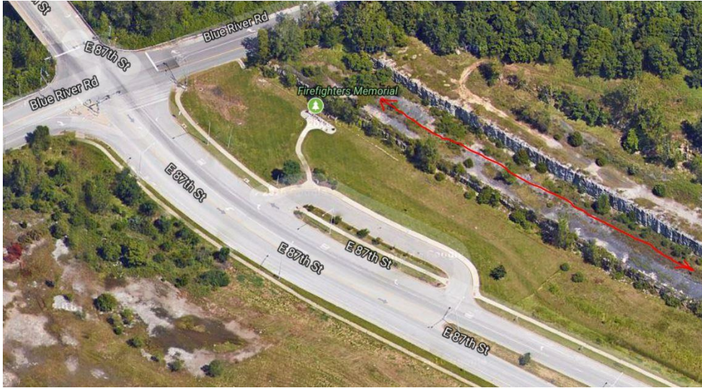
Figure 2.4. 87 th and Blue River Road section (87 th H) pointed with the red arrow.
