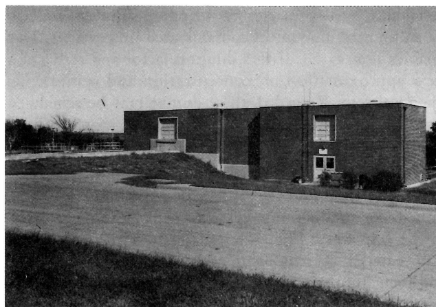
Fig. 4—Opposite side of control building for waste treatment plant.
