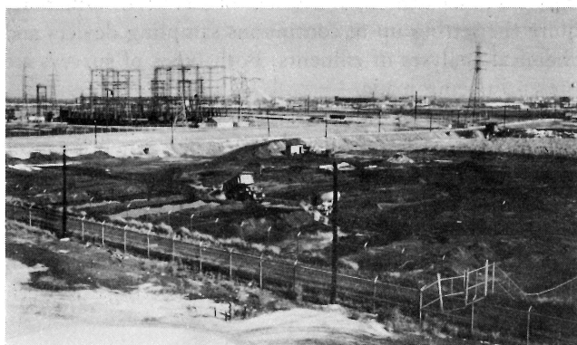
Fig. 2—Sanitary land fill used for disposing of tars and crystalline residues.
