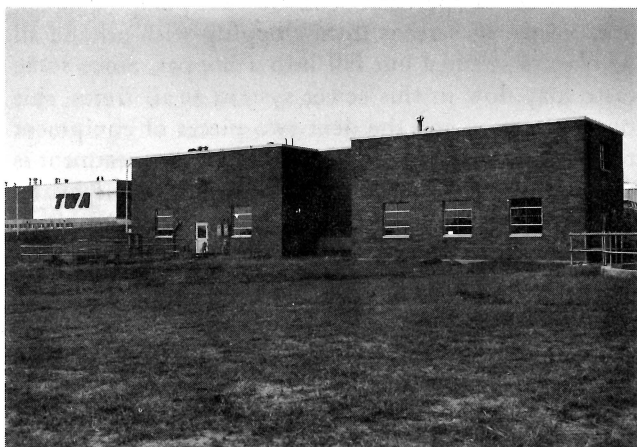
Fig. 3—Control building for waste treatment plant.
