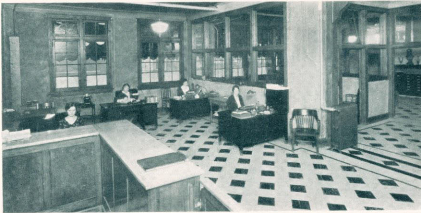
The administration office
