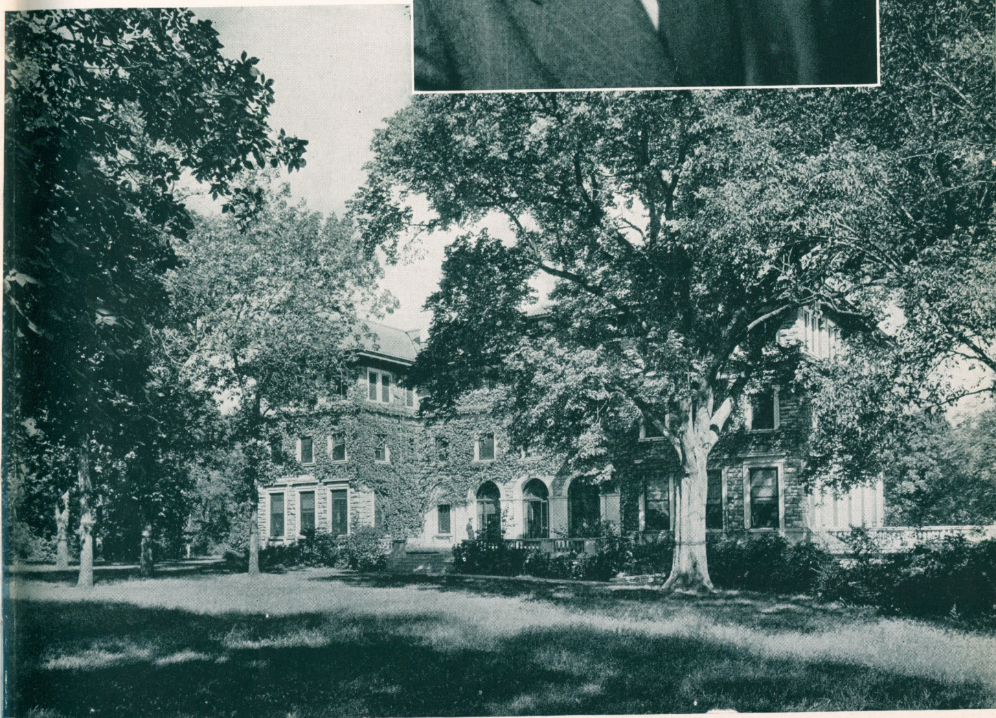
UNIVERSITY ADMINISTRATION BUILDING
