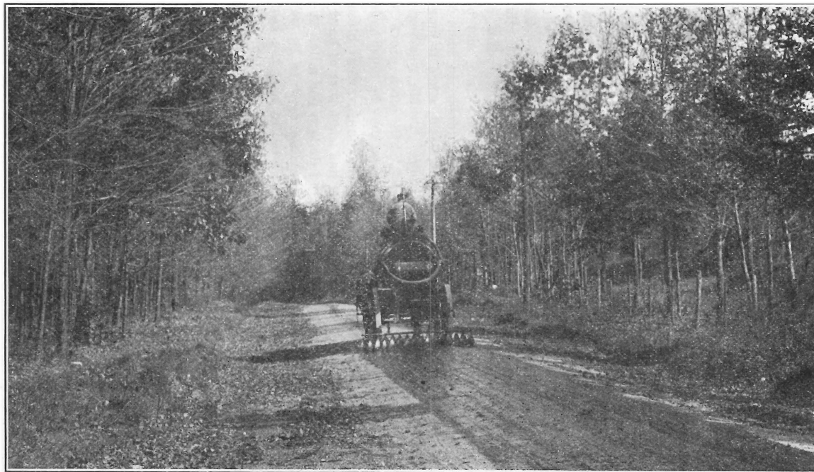
Fig. 1. Surface Oiling of Road
