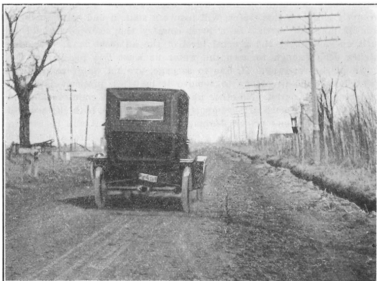
Fig. 4. Showing Crowned Roadway with Side Ditches Open
