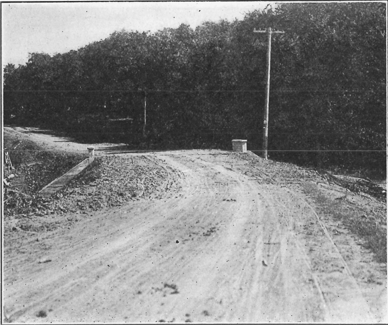
Fig. 3. Small Culvert with End Walls
