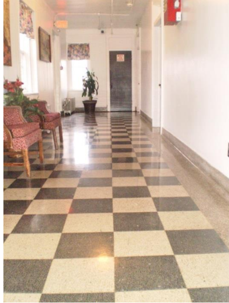
Figure 31. Bridgemont, second floor corridor
