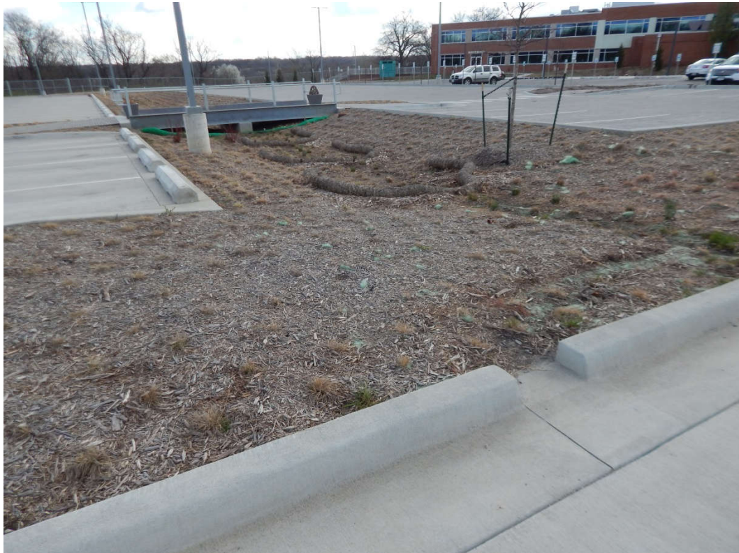
Figure 2.7.3: Curb Cut at KCMO Water Services Building
