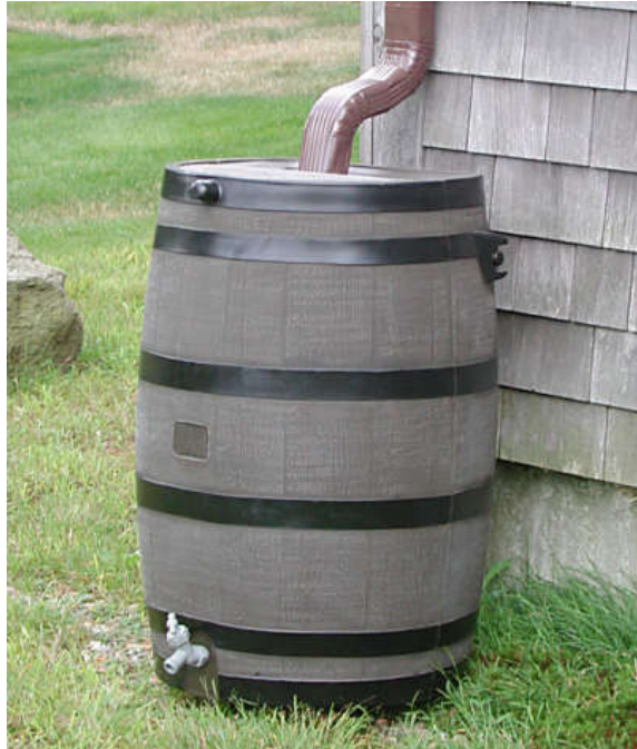
Figure 2.7.7: Typical Rain Barrel (Source: City of Barberton, Ohio)
