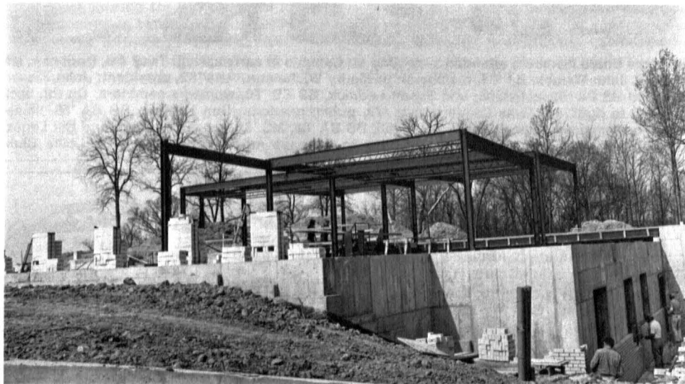
About 1,000 alumni and friends have contributed for the new Alumni Center, now under construction on Stadium Boulevard (740). Funds are still needed for the furnishings and office equipment.
