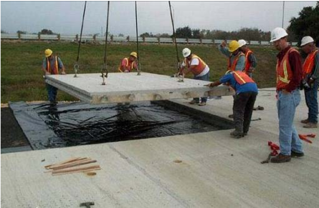
Figure 2.3 – Partial width panel placement on Georgetown Frontage Road, TX PPCP (Merritt 2002)
