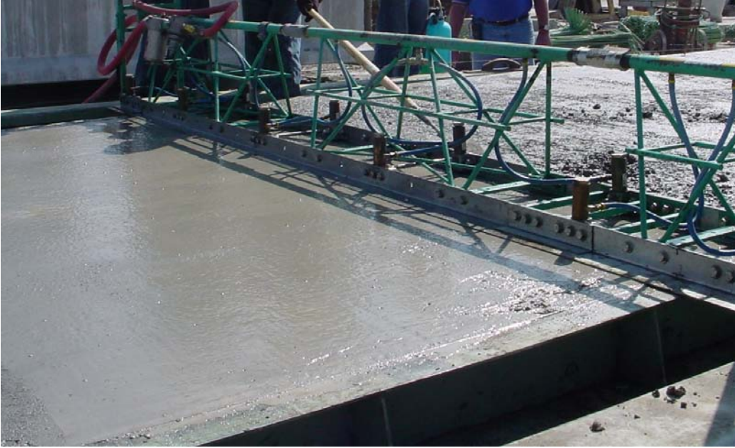
Figure 2.2 – Surface finishing of a typical base panel at the precasting yard
