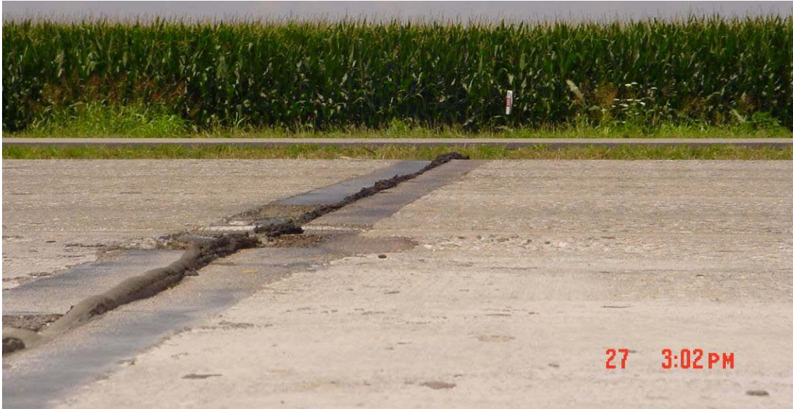
Figure 4.23 – Flexible joint compound squeezing out on a hot day with minor amount of chipping of rigid compound, Joint Panel A32 (June 27, 2006)
