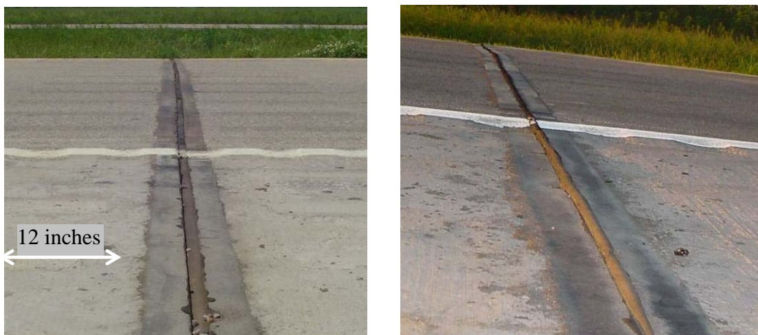
Figure 4.5 – Joint Panel A31 during mild temperatures (Left) and hot temperatures (Right)
