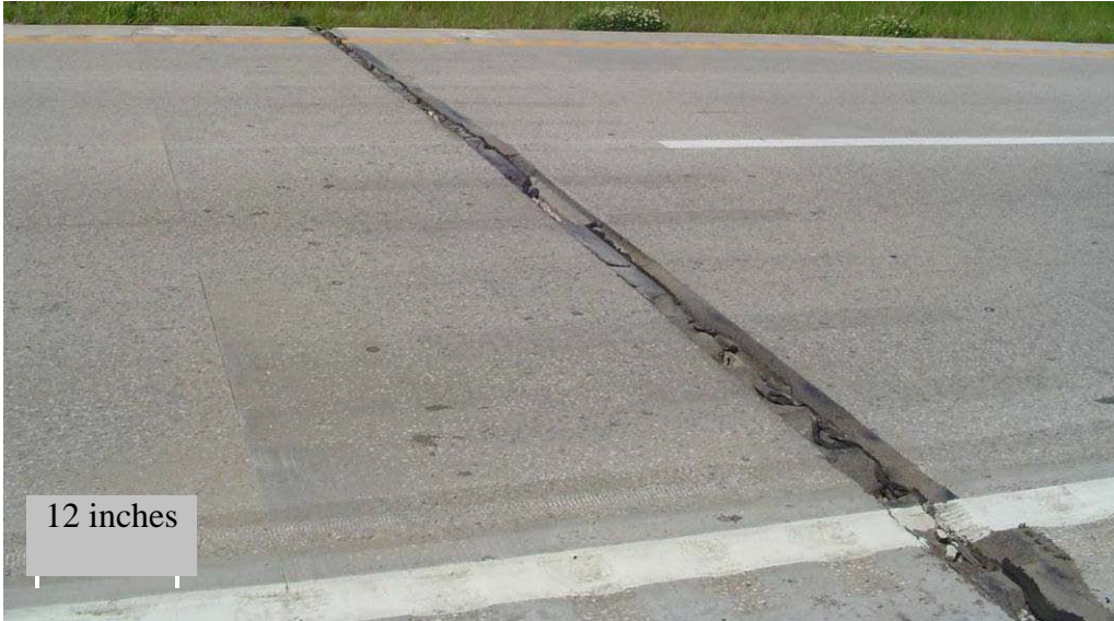
Figure 4.25 – Moderate degradation to rigid joint compound, Joint Panel A32 (May 9, 2007)
