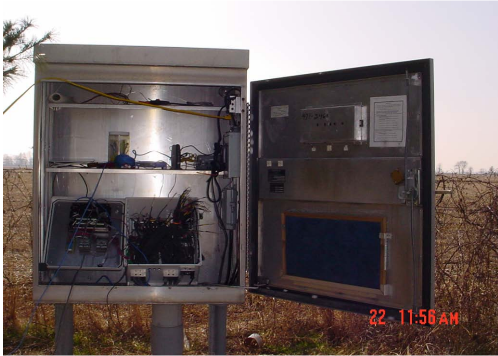
Figure 3.9 - Signal cabinet with main data-acquisition equipment installed at the edge of right of way
