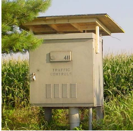
Figure 3.14 – Signal cabinet protected during the heat of the day by a shade roof
