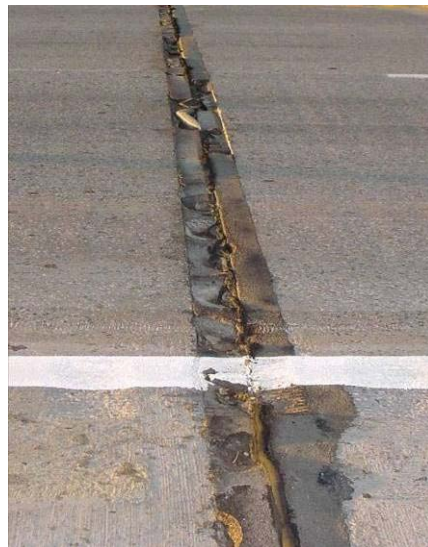
Figure 4.24 – Rigid joint compound chipped away more extensively, Joint Panel A32 (August 16, 2006)
