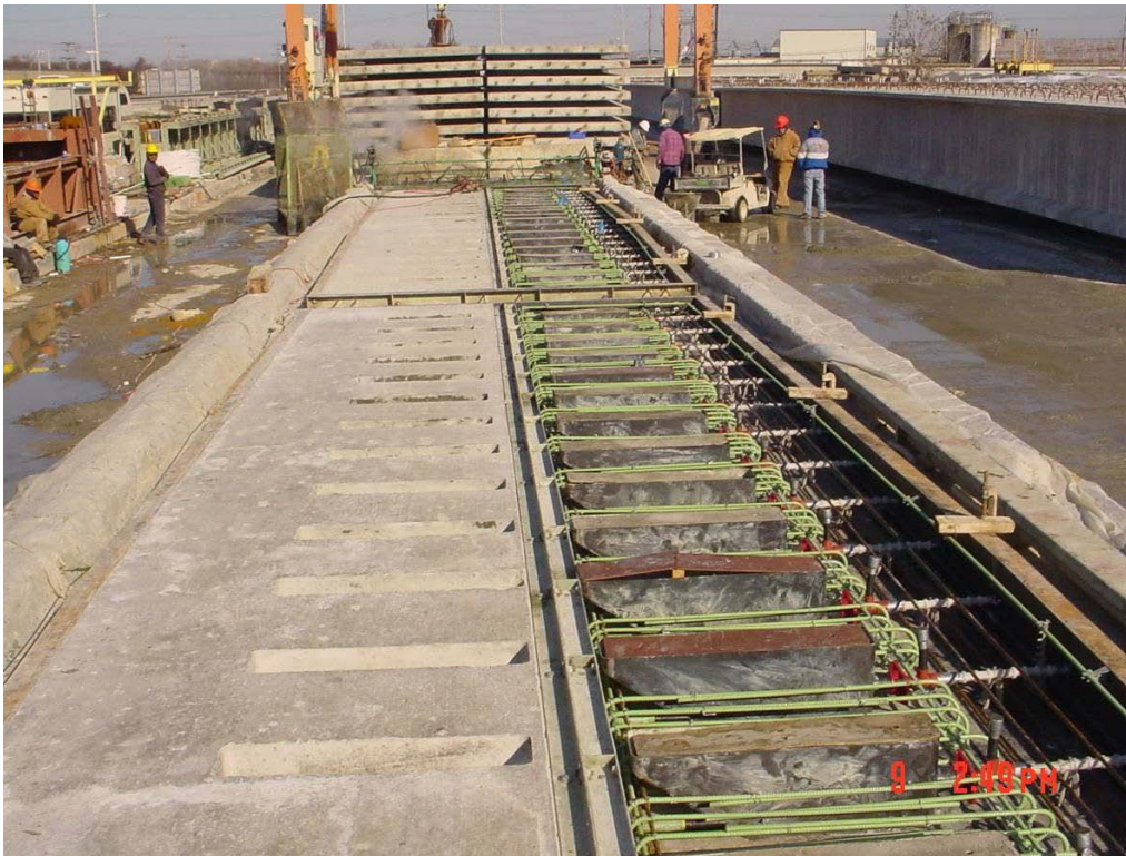
Figure 1.9 – Joint panel casting (left side cured for 1 night, right side ready for casting on 2nd day)
