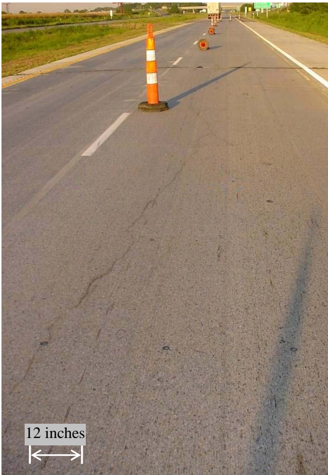
Figure 4.20 - Longitudinal crack in driver side wheel lane
