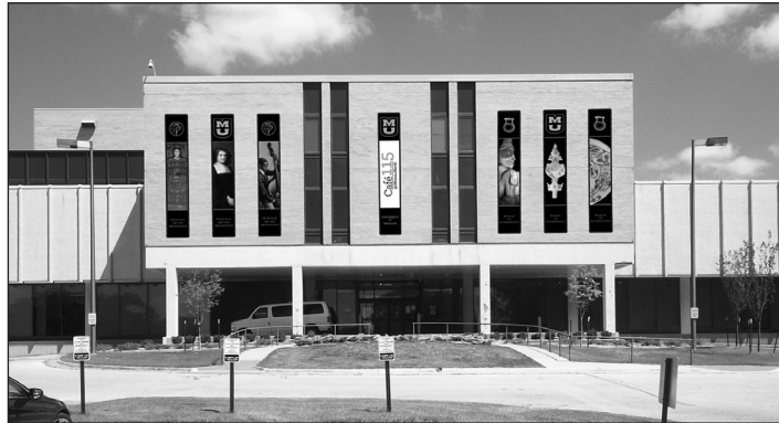
Fig. 2. Design for the south façade of the east wing of Mizzou North. Photo: Campus Facilities.
