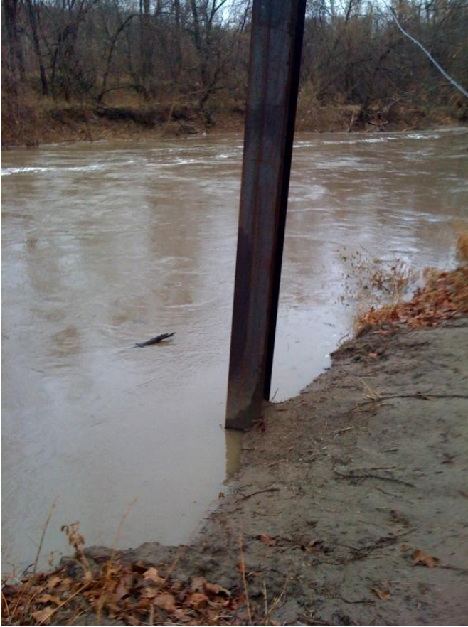
Figure 5-20. Photo of Pile during High Water Event, December 27, 2008.
