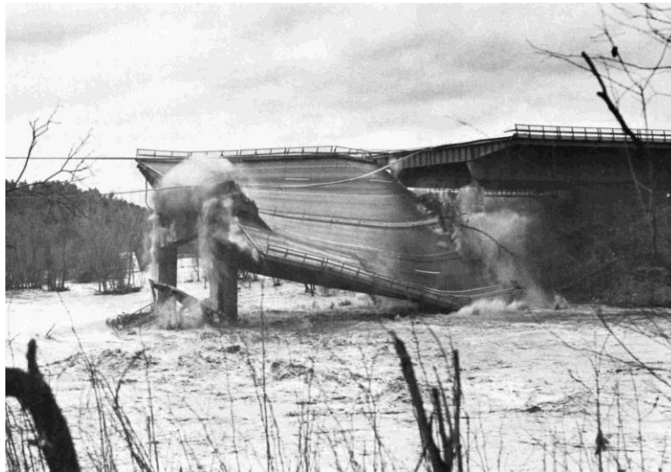
Figure 2-1. Photograph of the Schoharie Creek Bridge collapse, 1987.
