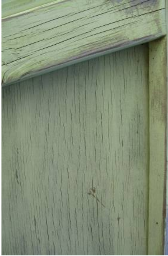
Figure 12. Ventilation System , detail, 2007.
