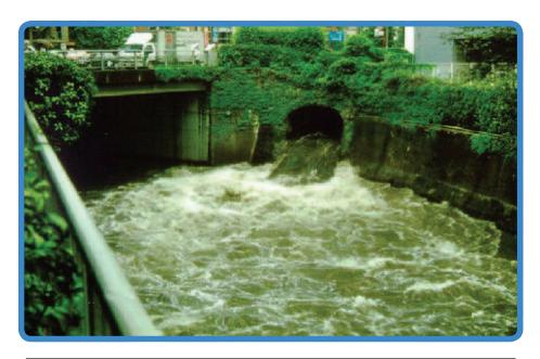
In a Combined Sewer System, water from industrial waste, home sewage, and rainwater runoff all flows into a single pipe.
