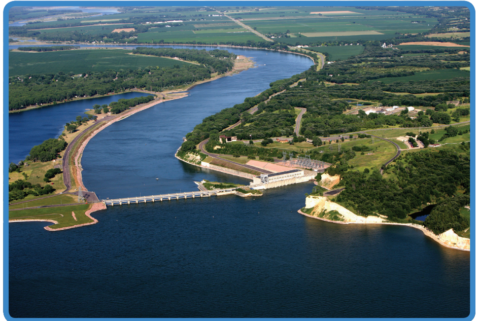
This is a downstream view of Gavins Point Dam and Lewis and Clark Lake, taken in 2008.
