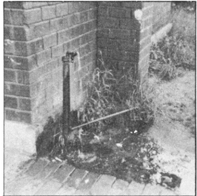
Fig. 65.—This is an inverted faucet at an athletic field which is used by the general public as a drinking fountain—the lip may easily be contaminated.
