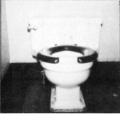
Fig. 35.—A water closet as an integral part of the school, submerged valve supply.
