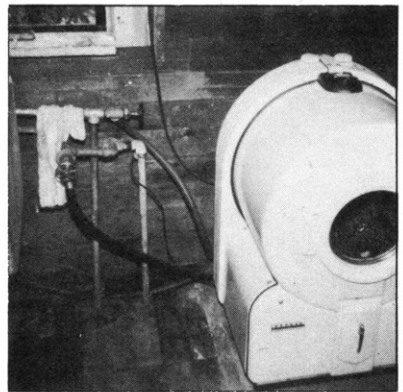
Figs. 49 and 50.—Two examples of Bendix washers with submerged water lines. Note the submerged hose supplies.
