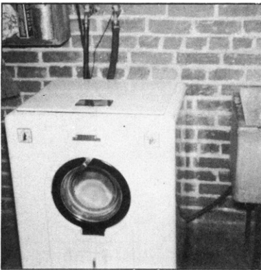
Figs. 49 and 50.—Two examples of Bendix washers with submerged water lines. Note the submerged hose supplies.
