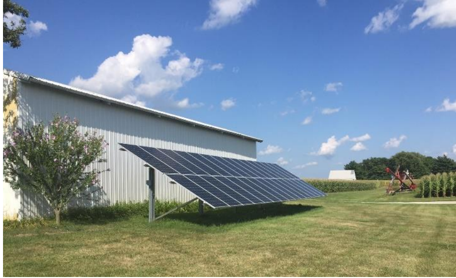
Image 10. The Farm Matriarch's ground mounted PV array
