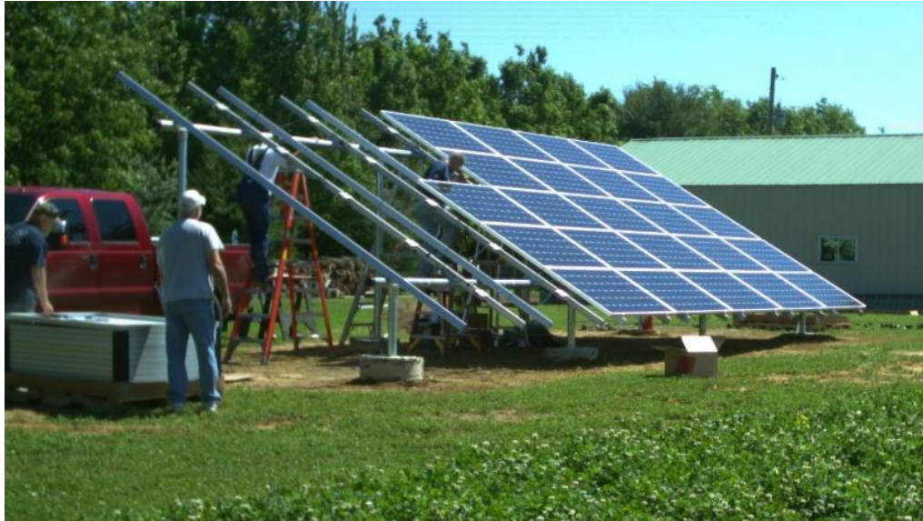
Image 5. The Firefighter's ground mounted PV array during installation
