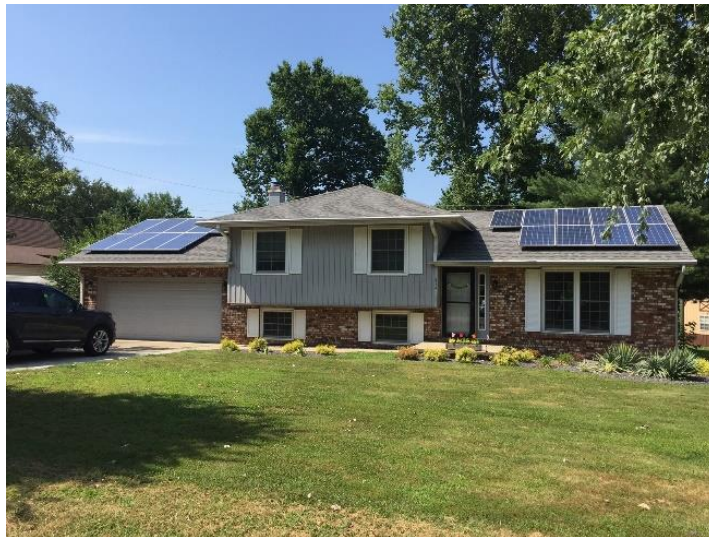
Image 8. The Energy Consultant's PV array
