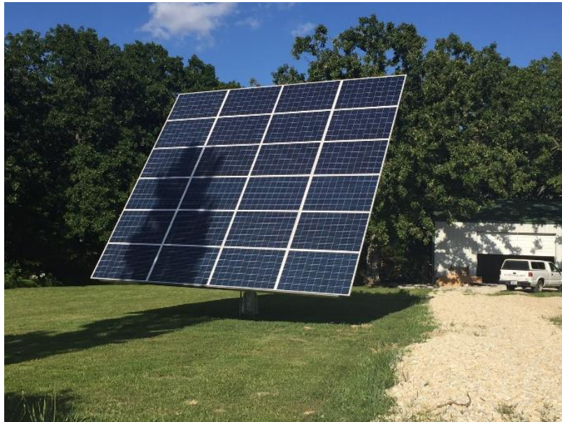
Image 14. The Young Adopter's PV array on a tracking system
