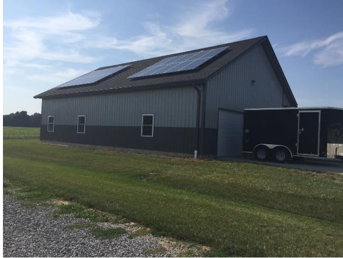
Image 9. An example of installation by the Energy Consultant
