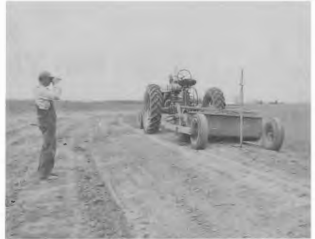
Fig. 14—Checking the height of a terrace ridge.
