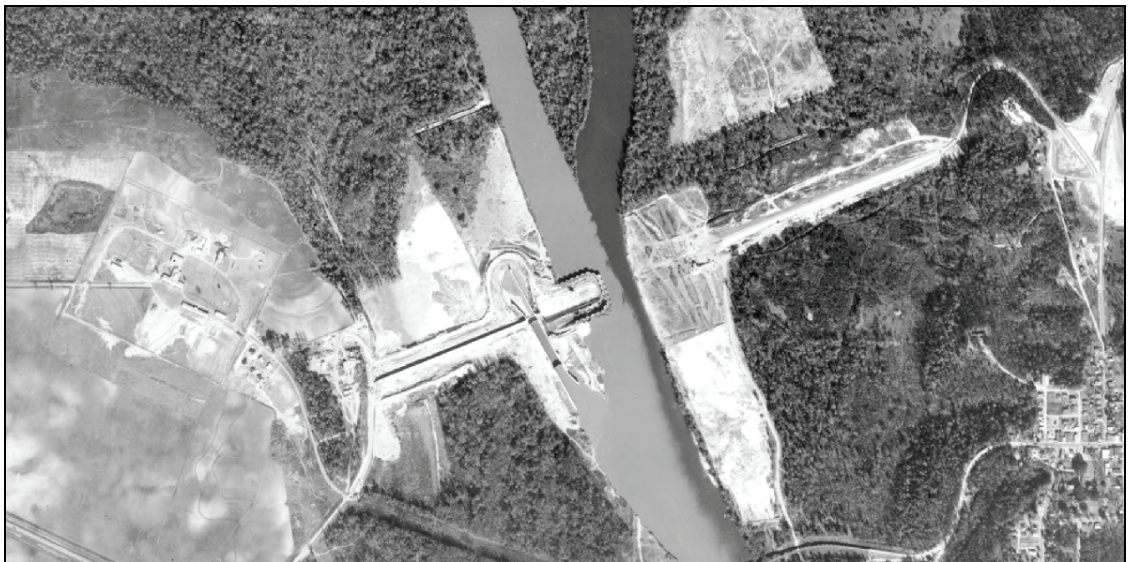
Figure 4. Aerial photograph of the Jim Woodruff Lock and Dam construction site in 1952 at the confluence of the Flint (right) and Chattahoochee (left) rivers (Agricultural Stabilization and Conservation Service Image LK-1M-031).
