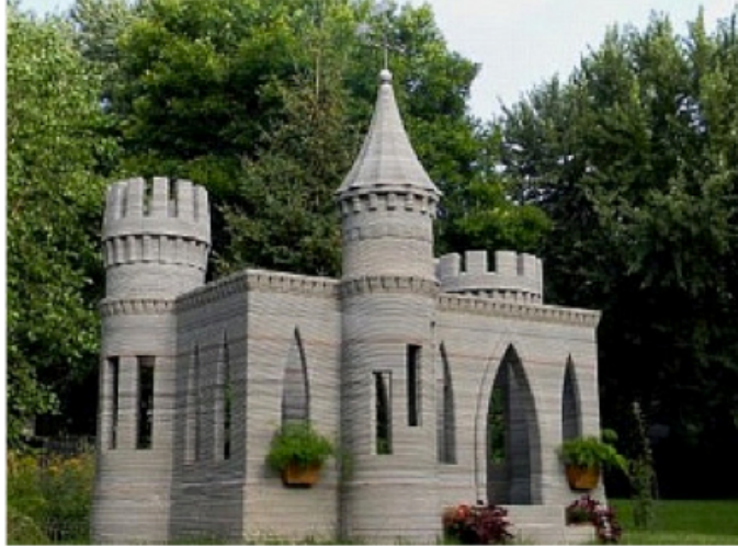
Figure 5 – Andy Rudenko’s concrete castle [9].
