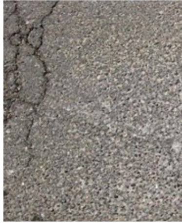
Figure 2.6: Mixed cracks.
