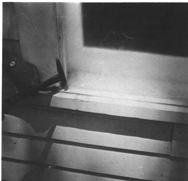
Use wooden strips with polyethylene storm windows to increase stability.
