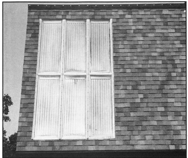
Six-panel array, 72 square feet net area, installed flush in the roof.
