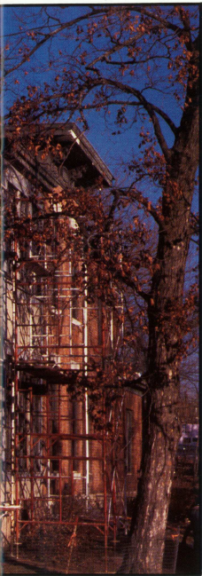
WORKERS REPAIR the deep bracketed eaves of the Conley House, an Italianate Revival Victorian style home built in the 1860s and located just southwest of Jesse Hall.
