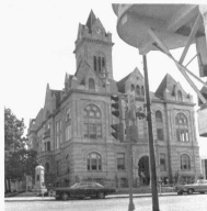
Cole County Courthouse, Jefferson City
