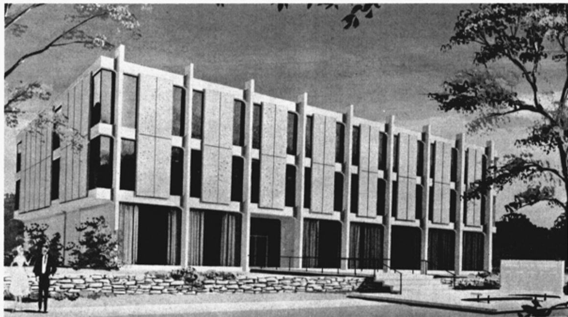
New Pharmacy Building is partly completed.
