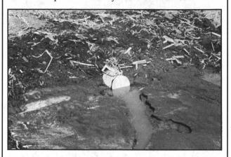
Excessive sedimentation or ponding of water at the outlet may restrict the water flow or cause a complete blockage if the water freezes. A blocked outlet increases the chance that the entire system will fail.
