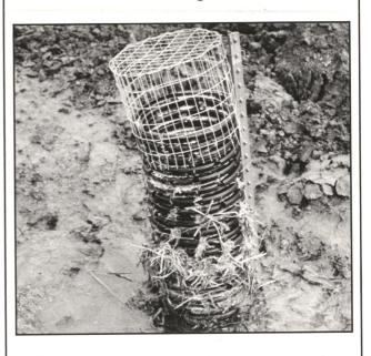
Install wire trash racks and caps to prevent trash from entering the conduit. Keep them in good repair and free of crop residue and other trash that reduce the flow. Control weeds with spot herbicide treatments. Weeds around inlets can restrict the flow and catch silt, and this causes wet areas in the terrace channel.
