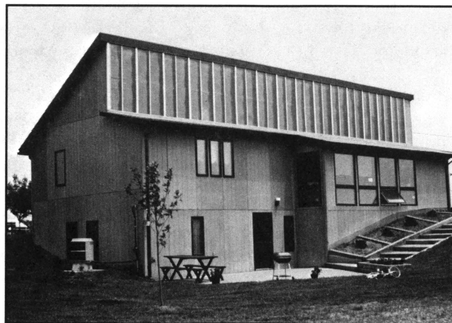
South view showing solar collector.
