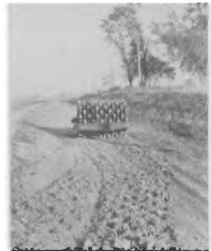
RIGHT—The sheepfoot roller; the tracks give an idea of the manner in which it compacts the subgrade.
