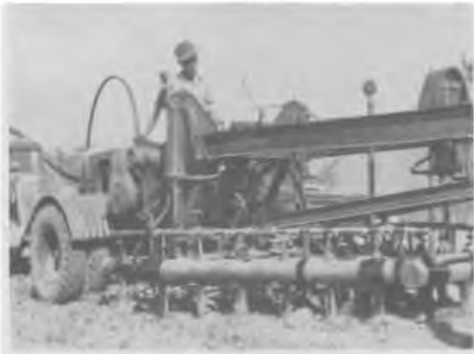
RIGHT—The sheepfoot roller; the tracks give an idea of the manner in which it compacts the subgrade.
