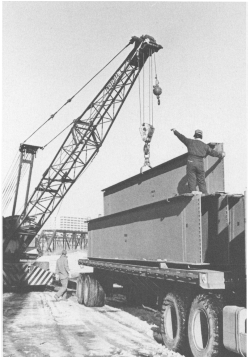
The 70-foot section of the old I-70 West bridge is lifted onto a truck to go first to Mosher Steel Company in Kansas City, Kansas for some fabrication work, then to Columbia.
