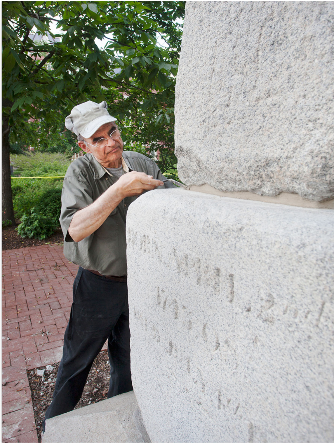
Robert Marti of Russell-Marti Conservation Services tuck-points a joint in the marble obelisk after it was reoriented. The granite is so coarse that, after Jefferson's death, detailed lettering could not be cut into the surface. Instead, his epitaph was carved into the marble tablet and attached. Photo by Rob Hill.
