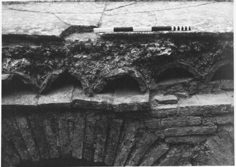
5. West Baths, Room 6, detail of floor construction.
